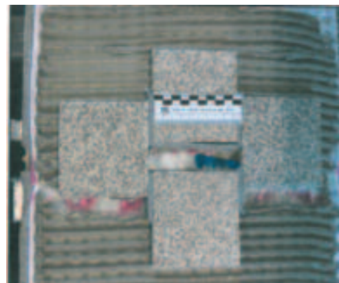
Crack widening and total rupture of decoupling
